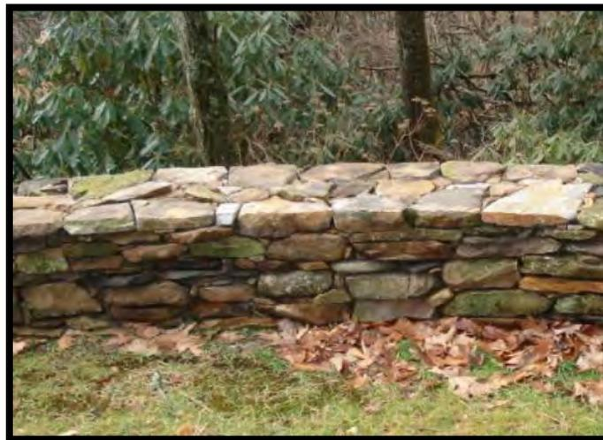
**Retaining Wall** – they can be decorative, but their purpose is typically structural and for the purpose of retaining steep slopes.
